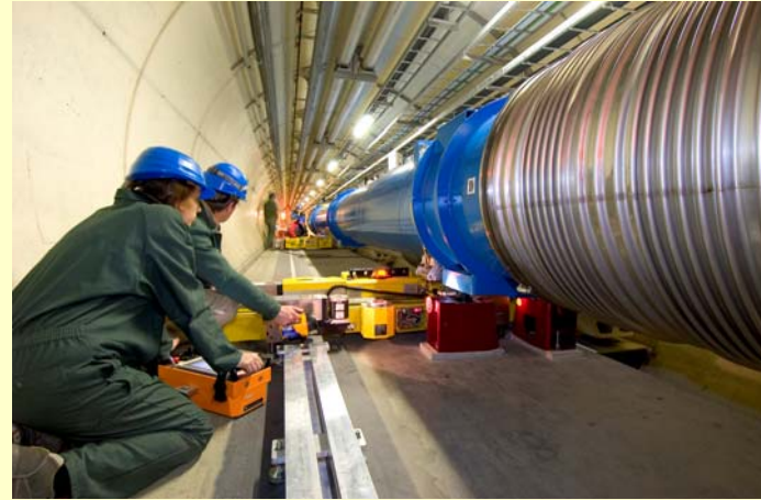
Installation work, underground
