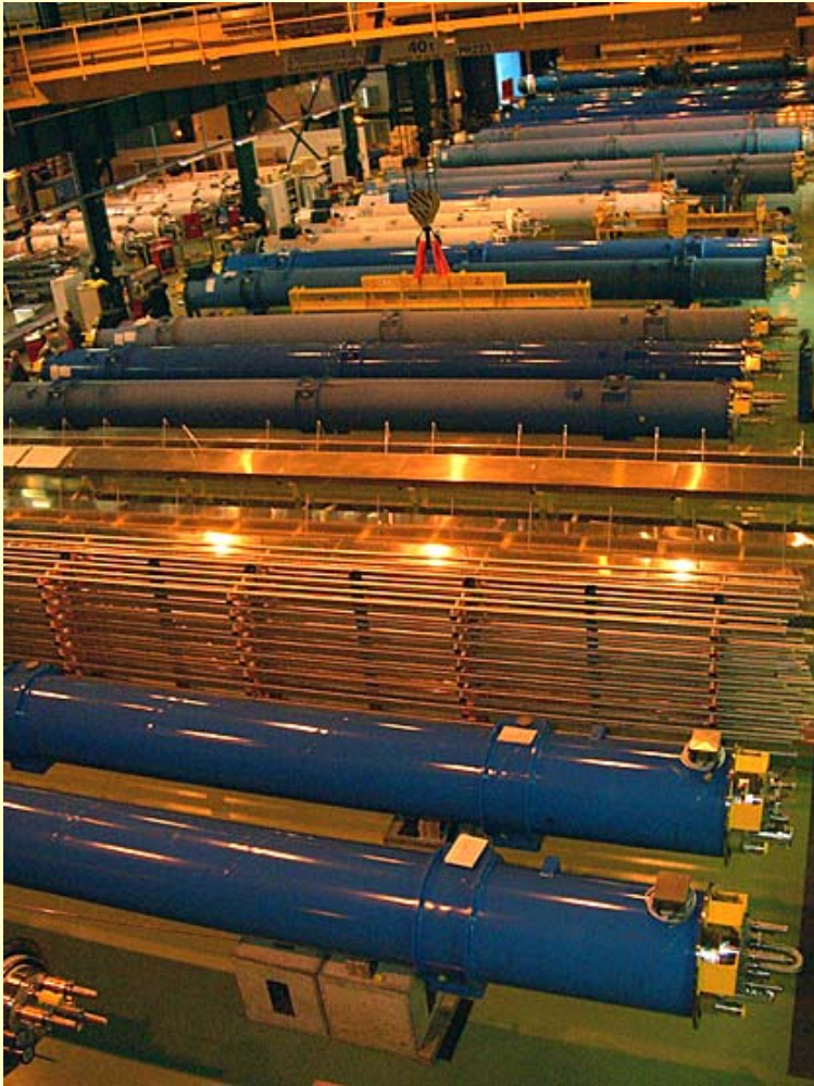
Preparation for installation, Hall SMI2
