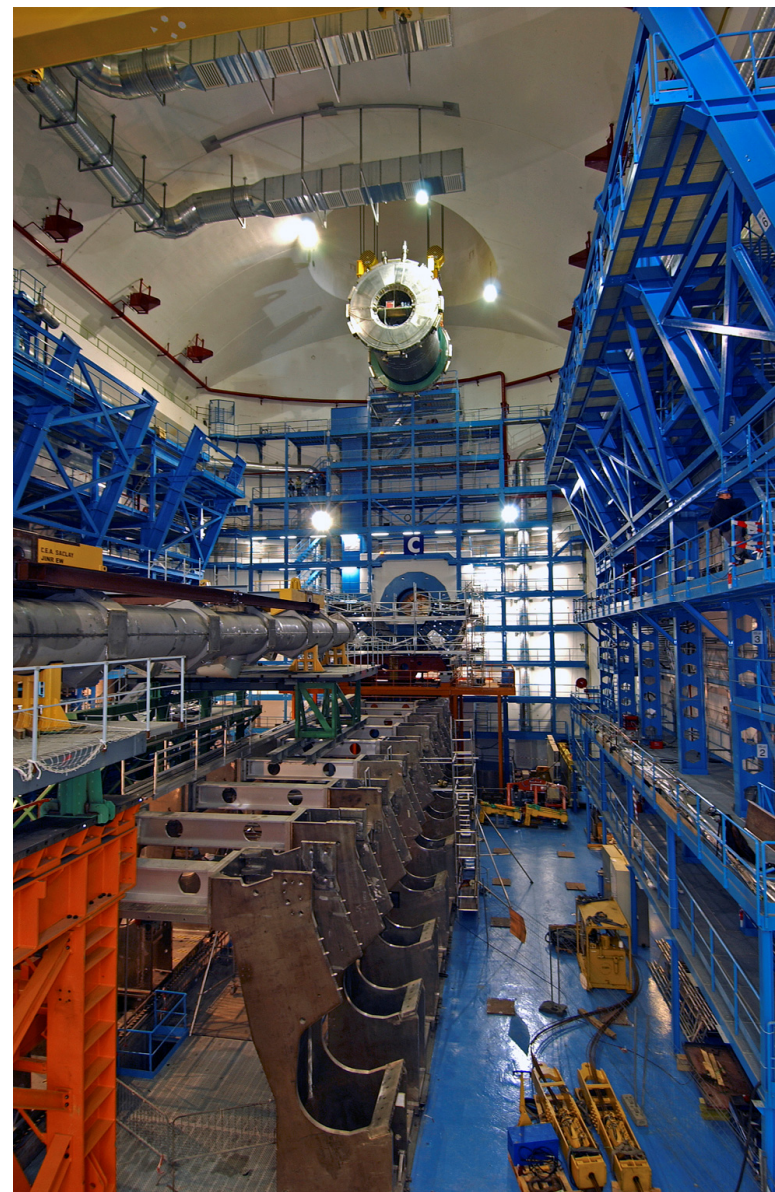
Transportation of Barrel LAr + Solenoid from Bldg 180 to ATLAS pit on Oct. 27 2004.
