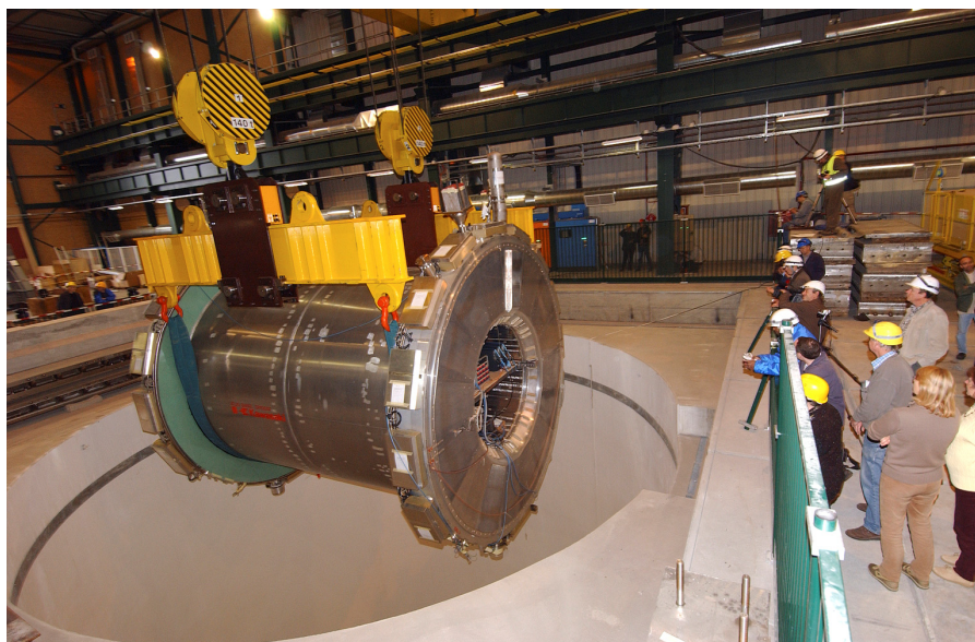
Transportation of Barrel LAr + Solenoid from Bldg 180 to ATLAS pit on Oct. 27 2004.
